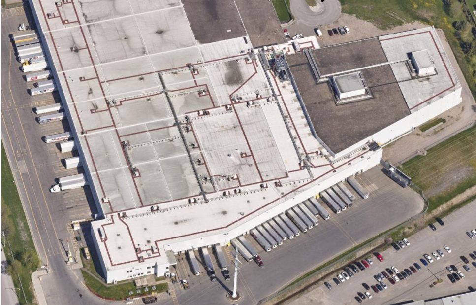
Centre de distribution Sobeys
